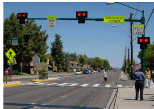
Figure 15. Pedestrian Hybrid Beacon
