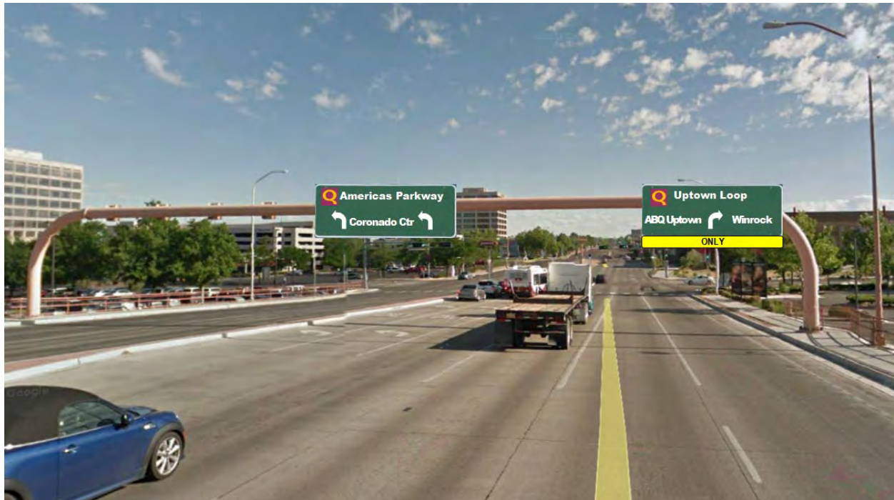
Figure 32. Overhead Destination Signs for Northbound Louisiana North of I-40
